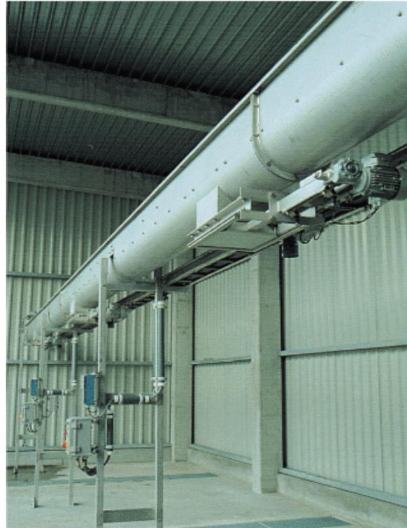
*A conveyor, 18.5 m in length, for the transport of dewatered sludge, Eeklo, Belgium.*
